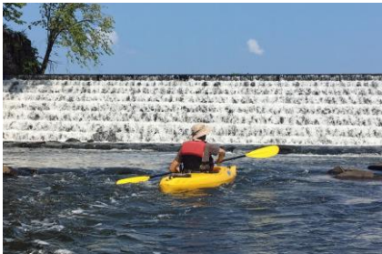
The stepped dam at Fisherville
