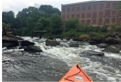
Portaging the broken dam
