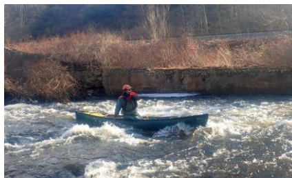
Jeff running the broken dam
