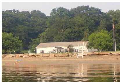
Cold Spring Community Center at the North Kingstown Town Beach
