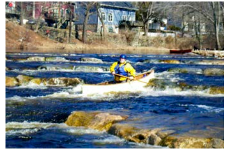
Jim C. running the drops in the new Kenyon Dam fish ramp.
